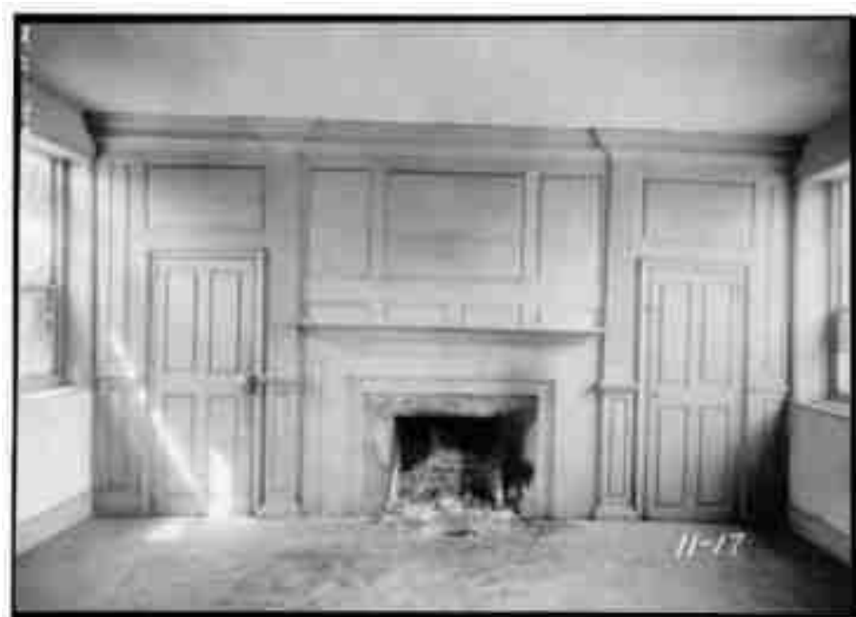
5. Interior, 1937, with pine paneling and closets flanking the fireplace, from 1936 HABS report
