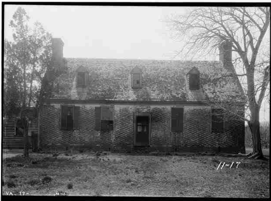
4. Main (east) façade, 1934, showing wood addition to the south, from 1936 HABS report
